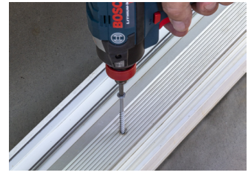
Sliding door track installation
